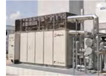
Fuel Cell in FR4 IBX in Frankfurt produces approximately 800,000 kilowatt hours of electricity annually.
